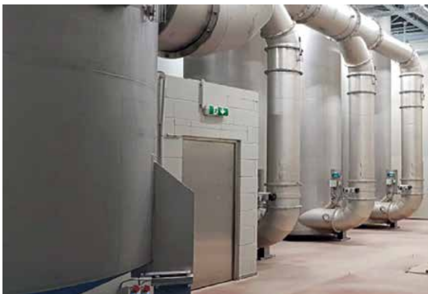
The three KMA electrostatic precipitators (right) and the gas scrubber (front left) ensure clean air quality compliant with TA Luft.
